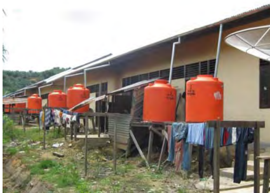
Plate 4: Newly Constructed Worker Housing with Tanks installed for Rainwater Harvesting
