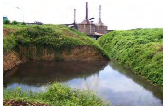
Plate 1: Pond for Treatment of EFB Stockpile Drainage
