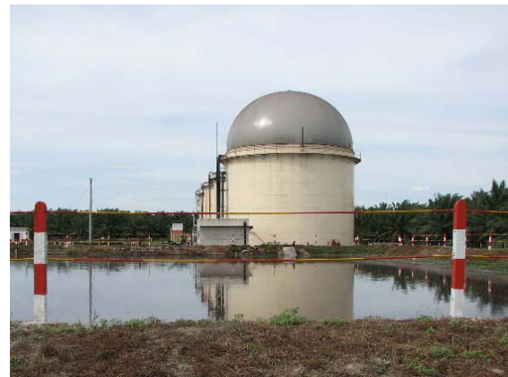
Plate 1: Mill Effluent Treatment Plant and Biogas Project
